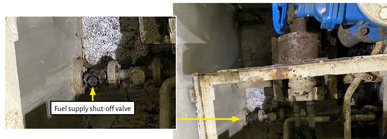
Figure: Fuel supply shut-off valve
