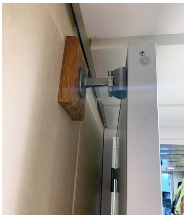
Figure 1: The hold-open mechanism on the door
