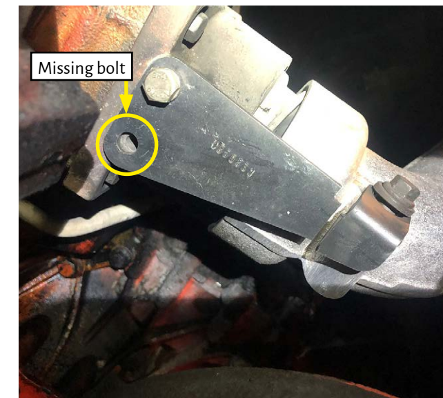
Figure 4: Fractured bracket and missing bolt
