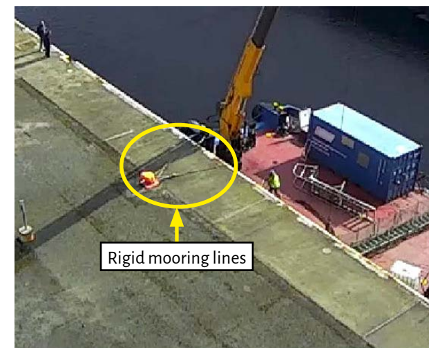
Figure 4: The workboat dropped in the lock and heeling over by 10°
