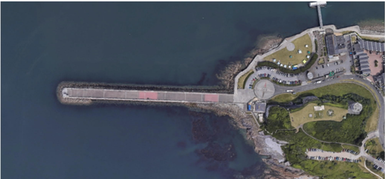
Figure 15.2: Mount Batten Breakwater
