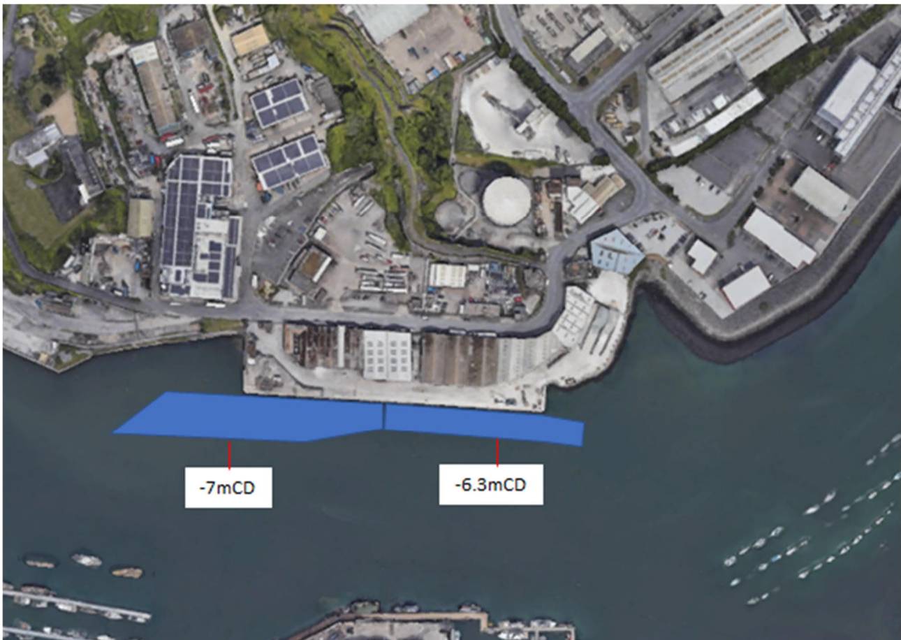
Figure 6.2: Cattedown Wharves Berthing Pocket
